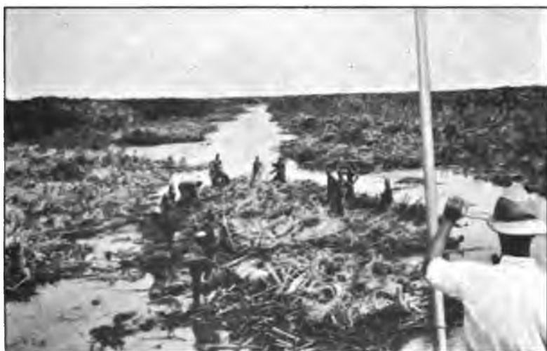
STEAMER TOWING OUT BLOCK OF SUDD: MEN STANDING ROUND AND HOLDING THE HAWSER IN POSITION.
