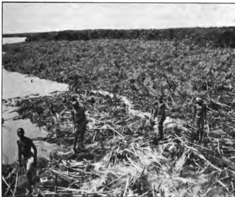
TOP GROWTH CUT DOWN AND BLOCK CUT INTO SECTIONS.
