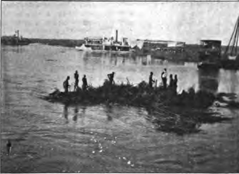
BLOCK TOWED OUT INTO OPEN WATER, MUCH DIMINISHED IN SIZE DURING ITS JOURNEY PARTLY BY COMPRESSION AND PARTLY BY THE FRONT EDGE ROLLING UNDER.
